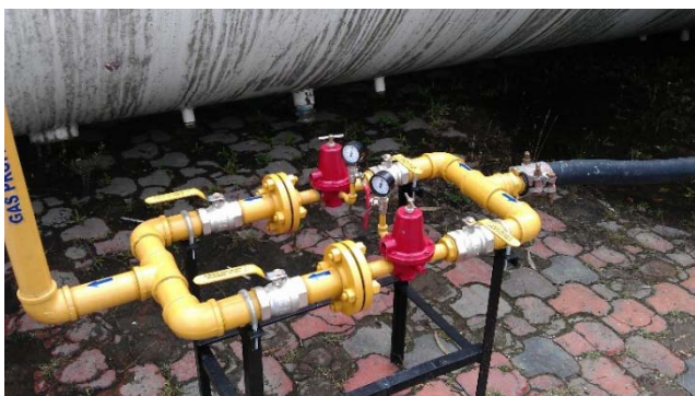
Figure 4: Tanker, lung tank and LPG supply bypass
