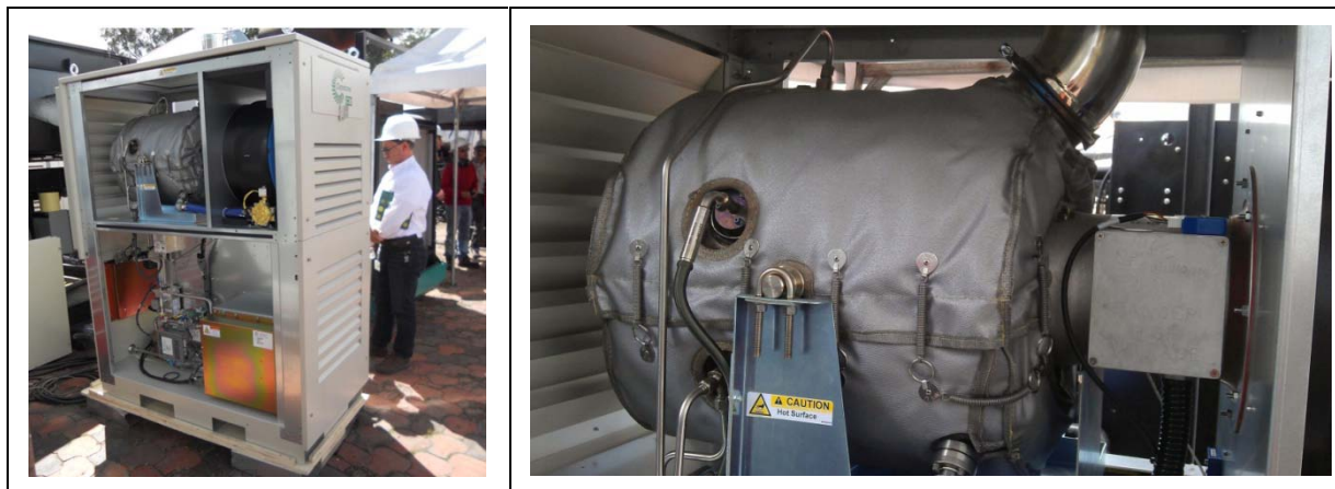
Figure 1: Location of the MTG at the Alsabana Campus test site
