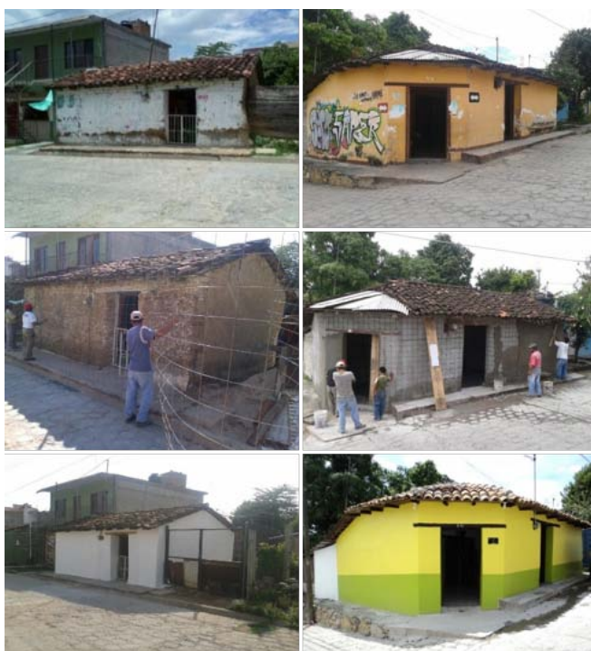
Image 13: Structural intervention in 2 adobe homes in Chiapa de Corzo
