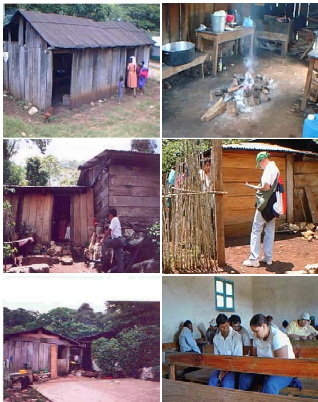
Image 4: Indigenous housing in precarious condition
