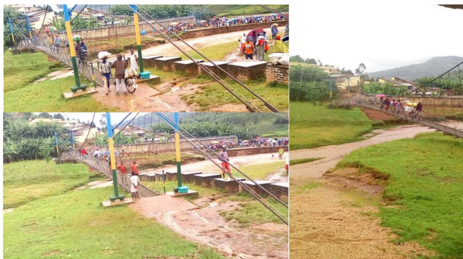
Figure 3: Community crossing the Gashyushya Pedestrian footbridge
