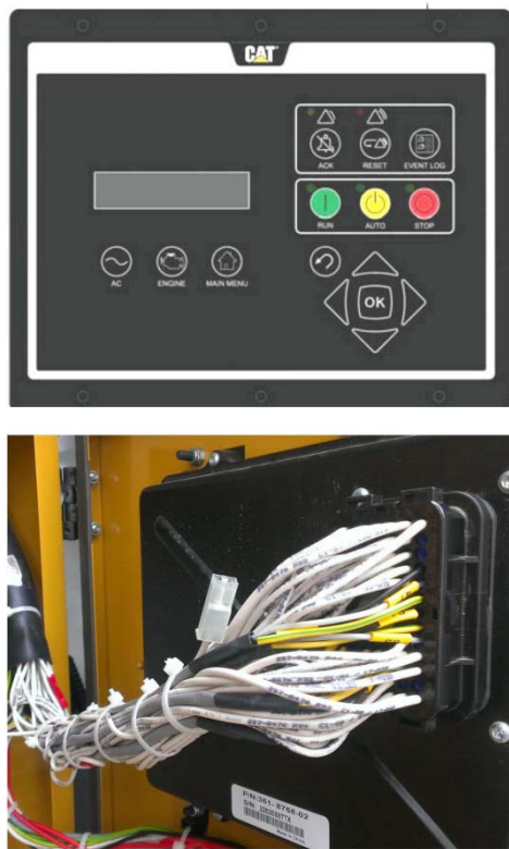
Fig. 3: Widely used DG controller, type EMCP 4
