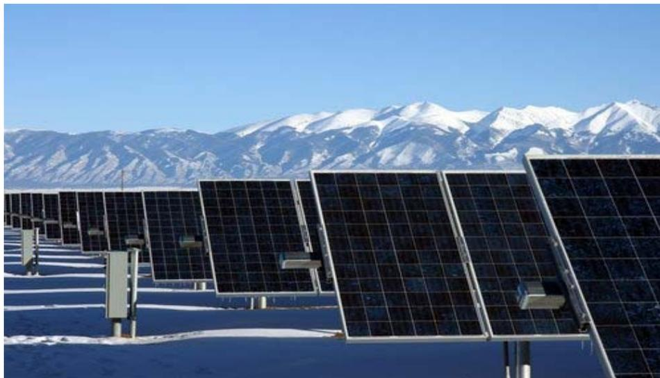
*Figure 14* : Seasonally adjusted fixed-axis photovoltaic panels at the Sun Edison photovoltaic power plant near Alamosa, Colorado
