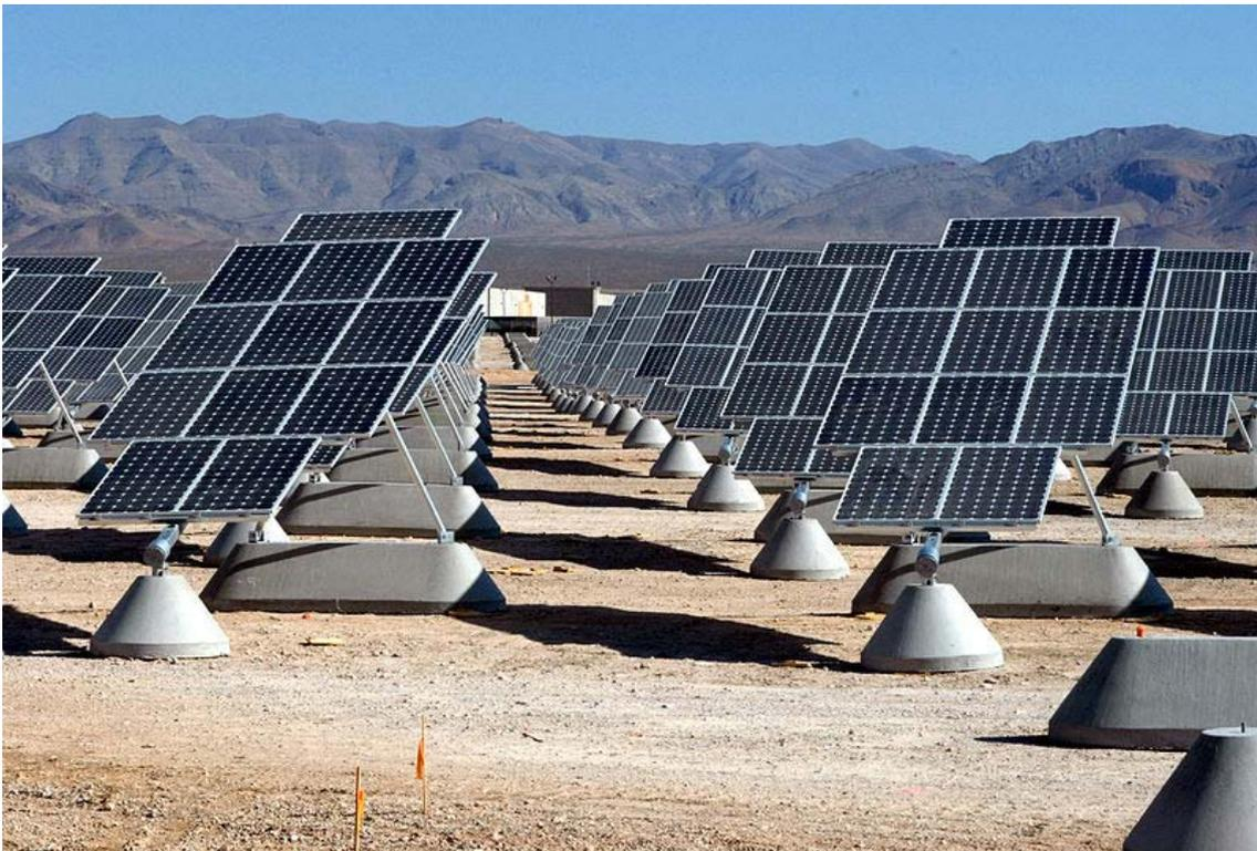
*Figure 17* : Single axis trackers with roughly 20 degree tilt at Nellis Air Force Base in Nevada, USA. The arrays form part of the Nellis Solar Power Plant. Credit: U.S. Air Force photo by Senior Airman Larry E. Reid Jr,
