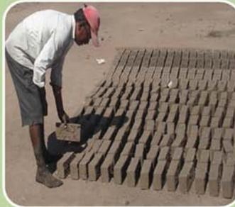
Bricks ' position is changed to dry the beneath area for 2 days
