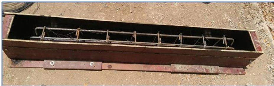
Fig. 3: Laying Reinforcement into wooden mould
