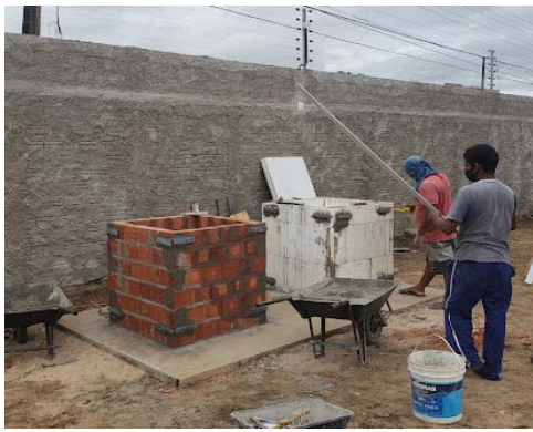
Figure 1: Prototypes under construction
