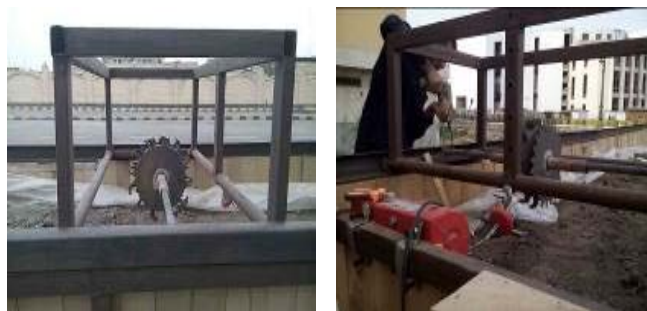
Figure 3: Attaching residue management unit on specified carriage for testing
