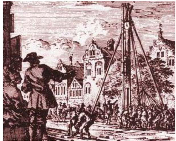
Figure 1 : Driving a pile. Picture by Jan Luyken (1649-1712)
