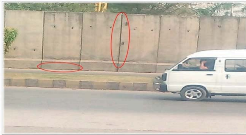
Figure 5: Weaknesses observed in existing arrangements
