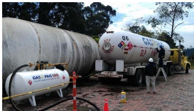
Figure 4: Tanker, lung tank and LPG supply bypass
