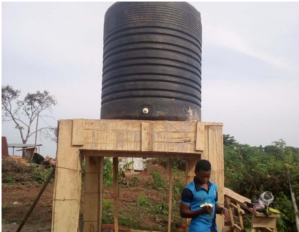
Plate 5: 3, 000 litres tank placed on the concrete platform
