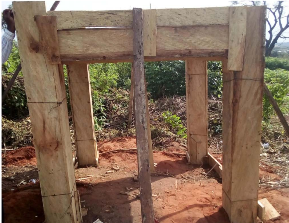
Plate 4: Form work prepared for the platform
