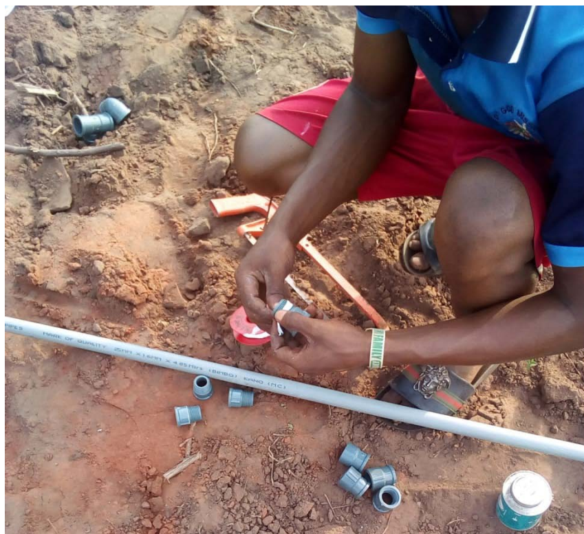
Plate 8: Installation of the emitting points and the perforated 1 inch pipe
