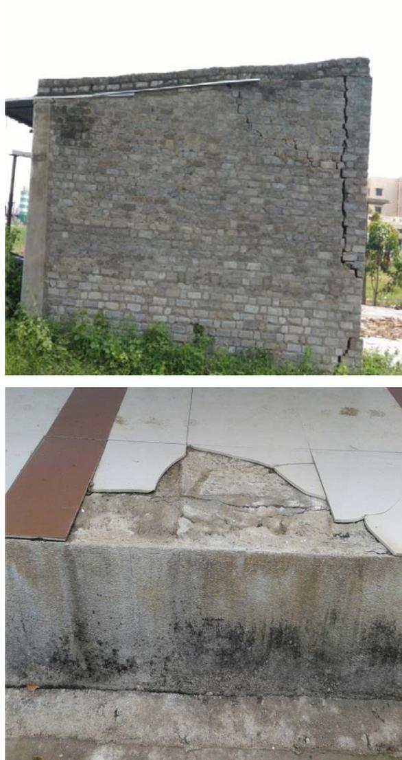
Figure 1 : Cracks, Swelling in Black cotton soil
