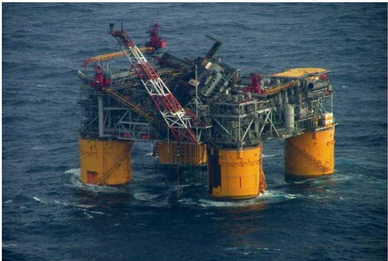
Figure 3 : Mars platform showing damage from Hurricane Katrina in 2005 (From [http://en.wikipedia.org/wiki/Mars\\_\(oil\\_platform\)](http://en.wikipedia.org/wiki/Mars_(oil_platform)))
