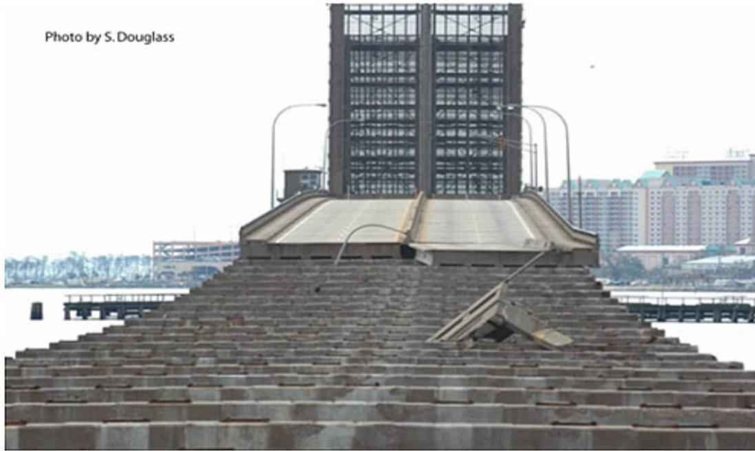
*Figure 5 :* US 90 bridge over Biloxi Bay, Mississippi was damaged by Katrina. Since the spans at higher elevations were not removed, the wave setup on top of the storm surge is more important than the wind loading (photo looking southwest from Ocean Springs 2/19/06, from FHWA-NHI-07-096)
