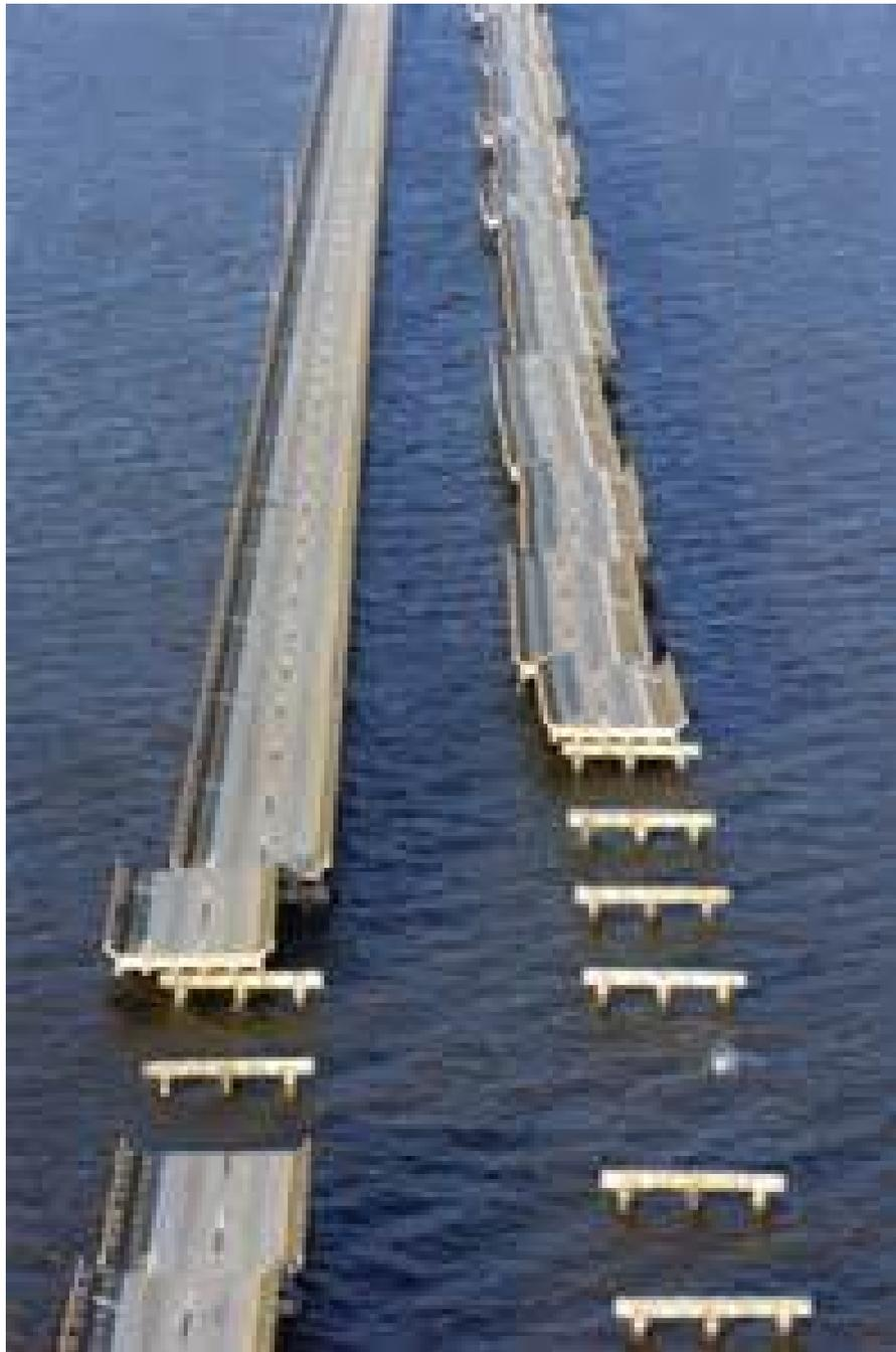
*Figure 4 :* Interstate I-10 over Mobile Bay damaged by Hurricane Ivan in 2004 (From FHWA-NHI-07-096). According to FHWA, the wave setup on top of the storm surge was the cause
