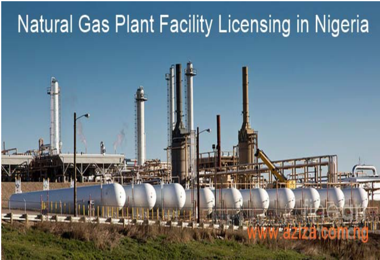
Fig. 1: Natural gas plant
