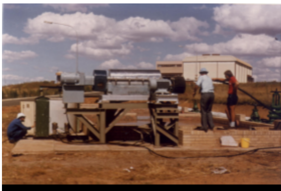
Figure 24: Sharples Polymizer 30000 centrifuge at the Saulspoor waterworks
