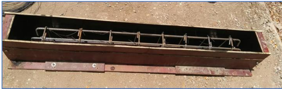
Fig. 3: Laying Reinforcement into wooden mould
