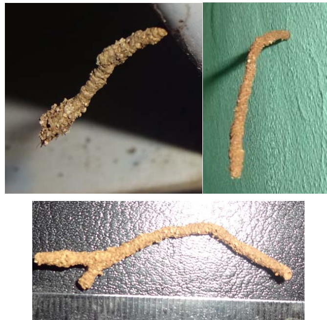
Fig. 10: Suspended mudtube over the concrete wall
