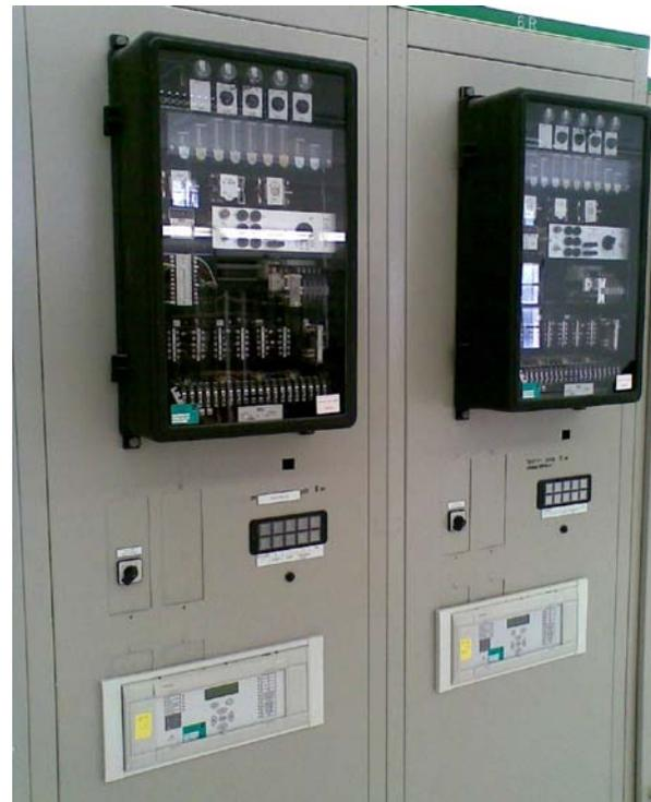
*Figure 2 :* Section of Distance Protection panel for critical 160 kV lines consisting of electromechanical relays type LZ31 (above) connected in-parallel with microprocessor-based protection MiCOM P437 (bottom)
