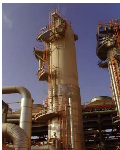
Figure 1 : The absorption packed column of In Salah Gas (ISG)
