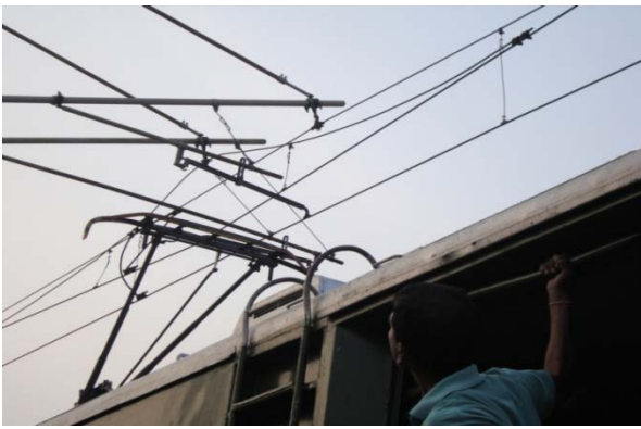
Fig. 2 : Testing of turn out OHE with Tower Wagon
