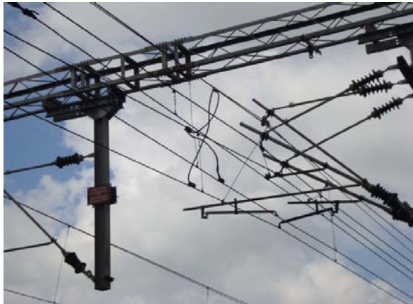
Fig. 3 : OHE Profile at Turn out Location
